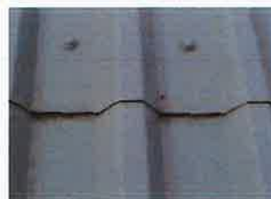
Colorcoat HPS200 Ultra® with Galvalloy® roof after 7 years.
