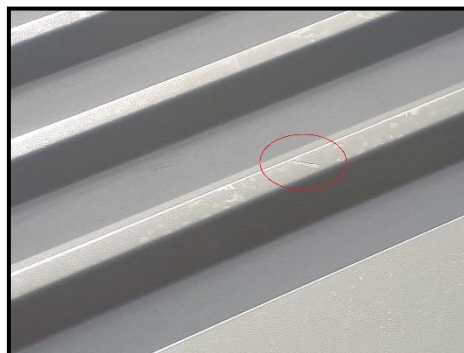
Image showing a scuff which has not penetrated the coating surface
