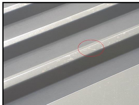
Image showing a scuff which has not penetrated the coating surface
