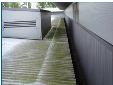
Image showing area of heavy deposits not cleaned by rain action
