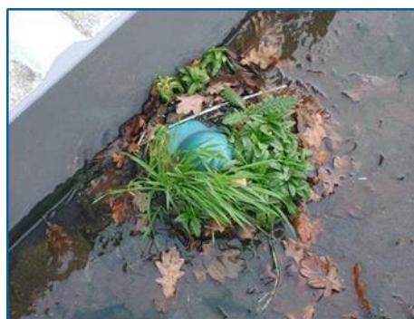
Buildup of organic matter around outlet that will effect performance
