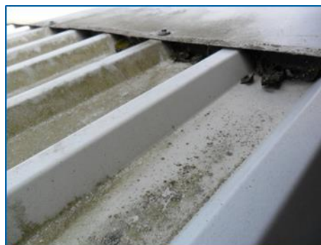
Image showing buildup of heavy deposits and detritus
