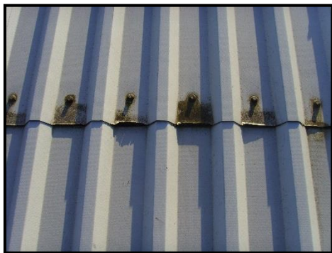
Image showing cut edge delamination
