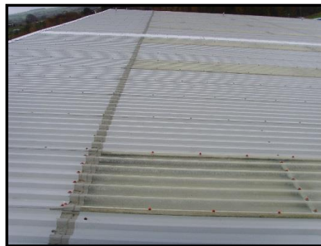
Image showing rectified cut edge delamination
