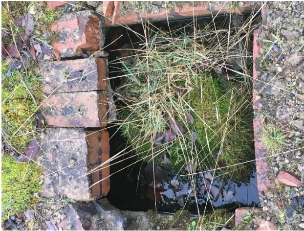
Photographs 7 Waterfilled manhole
